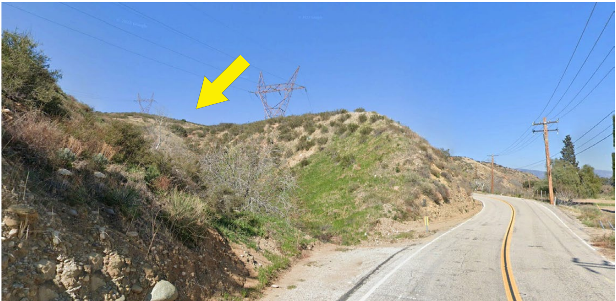
The view along Lytle Creek Rd. from the southwest corner of the site.
