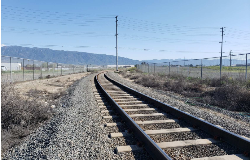
Photograph 5: View looking northeast at the BNSF railway that bisects the eastern and western parcels within the Project site.
